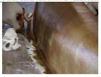
Trimming the excess fiberglass about an inch from the bottom of the wing tip
