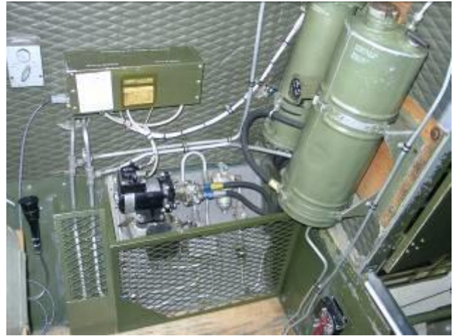
Hydraulic pump and reservoirs
