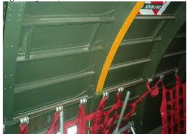
Seat Support Rail above the maximum inside diameter of the fuselage and showing intercostals between frames
