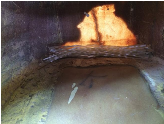
Fiberglass “unidirectional” fibers to reinforce the corner where the damage occurred
