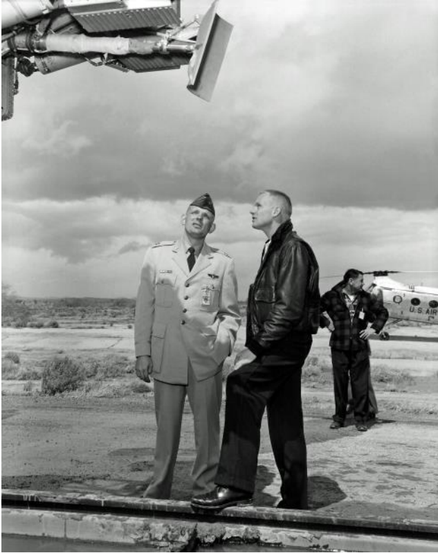
“Kinch” and new NACA pilot Neil Armstrong observe the X-15 ejection seat mounted on a rocket sled at the Edwards High-Speed Test Track. Supersonic sled runs verified that the life-saving seat worked as planned, although no pilot ever ejected from an X-15.
