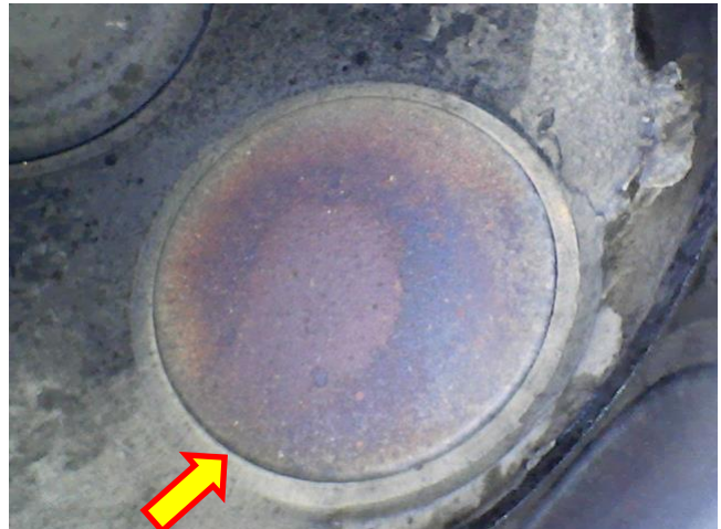
Cylinder #1 in 2020. Note brighter and cleaner appearance, which is not a good thing. Arrow shows where leak most likely was
