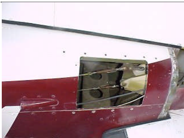
Completed access hole on left (port) side
