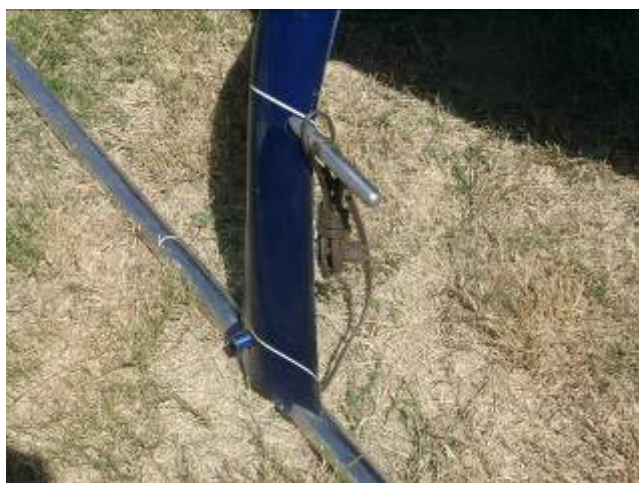
We would have thought the power cord would have been a larger cable. We hope the extension cord is strain relieved better than this picture would indicate.
